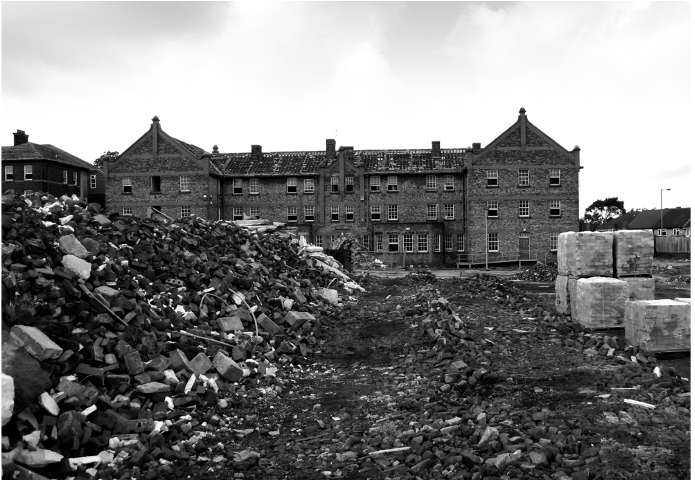
Demolition of the old hospital in 2017
