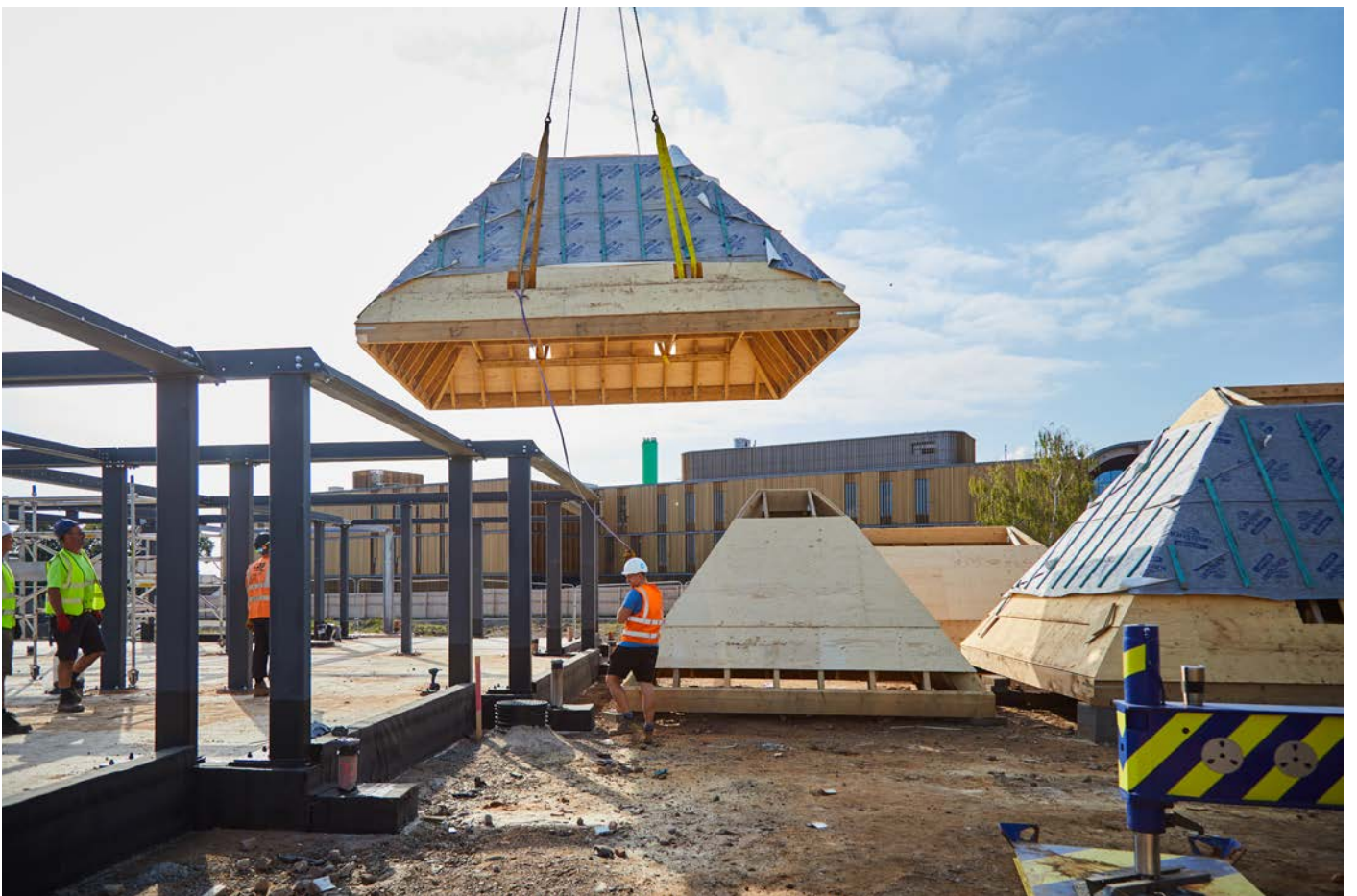
One of the roofs being lifted onto the steel frame
