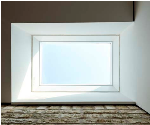
A skylight in the bathrooms
