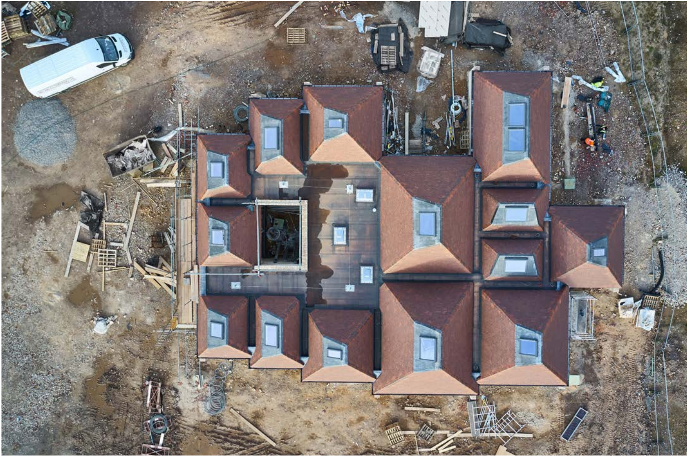
The view from above during construction
