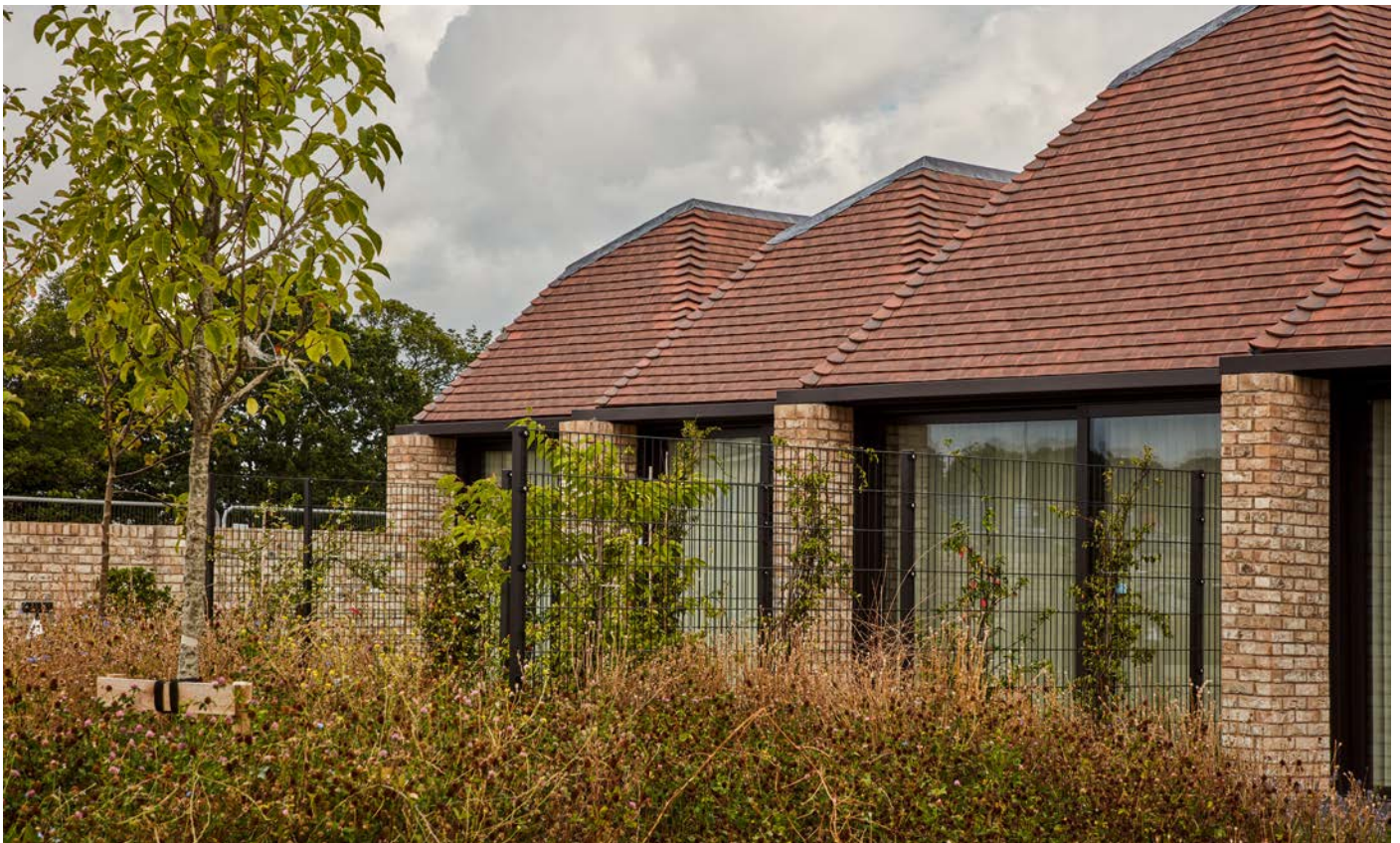
Staggered walls and planting provide privacy between counselling rooms.
